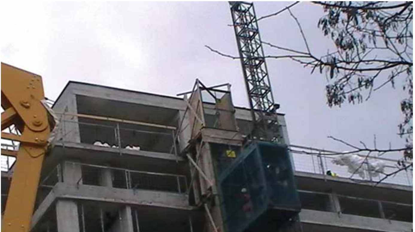
The top of the Ossington-Queen Street Rental Apartments, taken on March 1, 2012.
